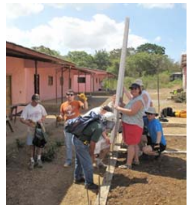
First wall panel goes up, March 28, 2011
